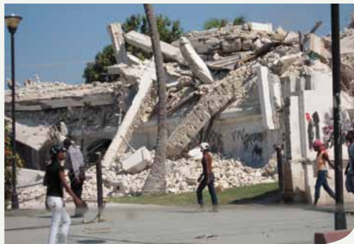
A building in Haiti after the earthquake in January
