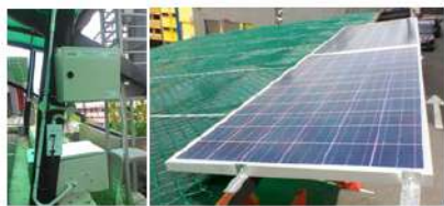
Figure 3: Installation of Solar Panel, Battery and Sensor to Car Park Structure
